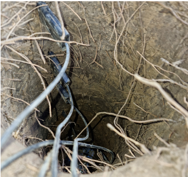
Soil moisture sensors installed in the rootzone
